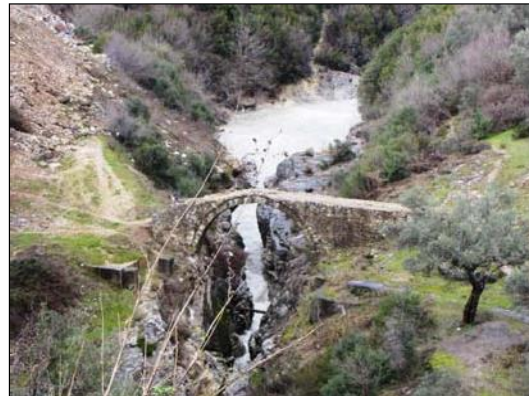
Figure 4 Old bridge of Brari Monument of Culture
