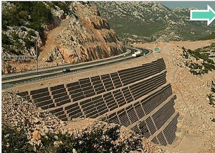
Gabion Retaining Wall in Highway (Bolu Mountain Highway ,Tekno Maccaferri Web Site, 2005)
