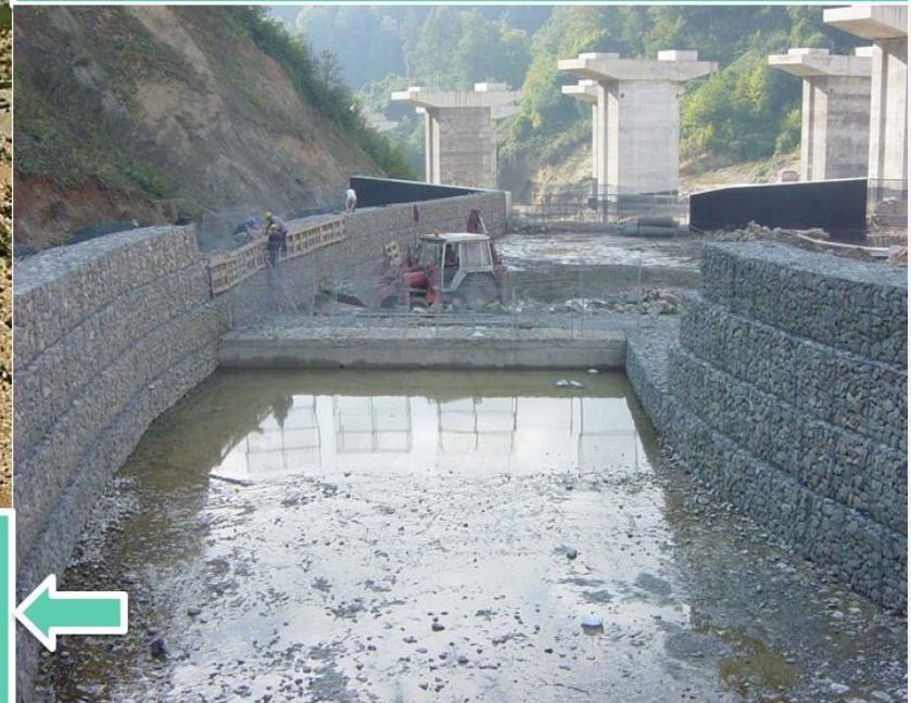
Gabion Retaining Wall (Wikipedia, Croatia, 2009)
