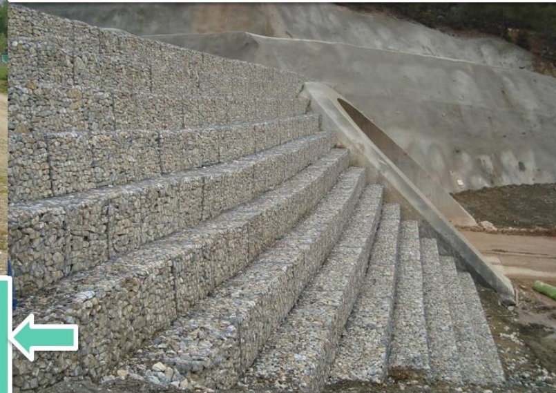
Western Black Sea Mattress Gabion in Stream bed improvement (Tekno Maccaferri Web Site, 2005)
